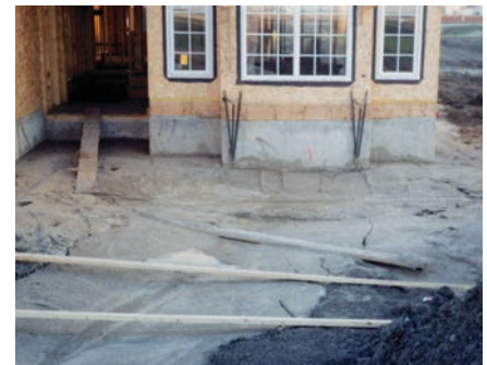
ABOVE: Liquid Backfilled foundations will provide a maintenance-free stable grade and a dry basement.
