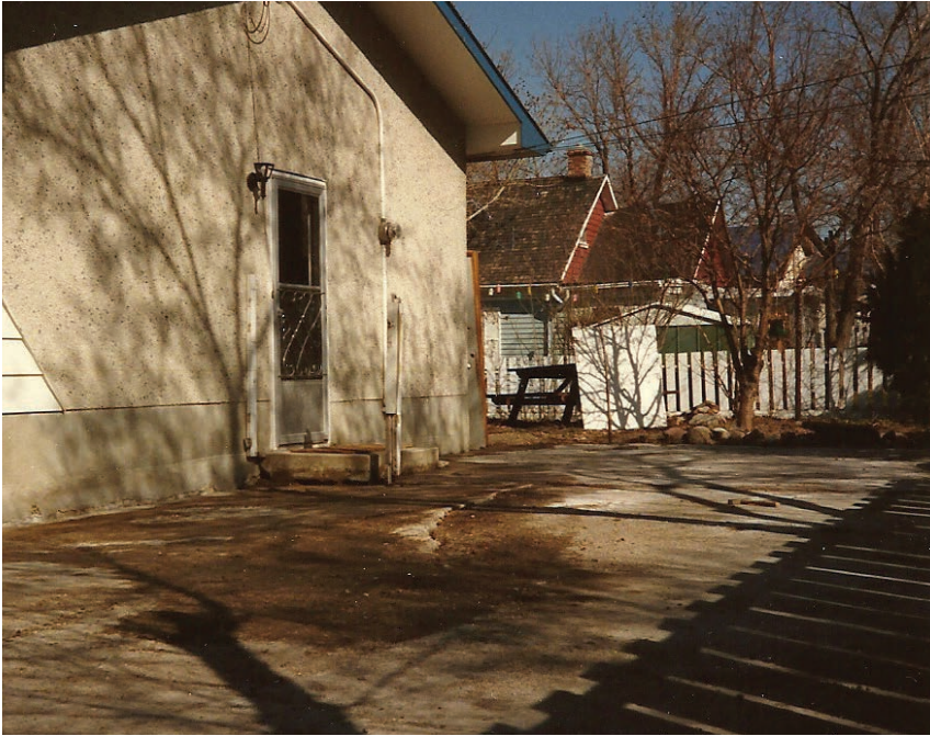
ABOVE: These settlement problems were caused by improper foundation backfill. The settled driveways above are in the process of being mudjacked up as much as 18 inches back to their original elevation.
