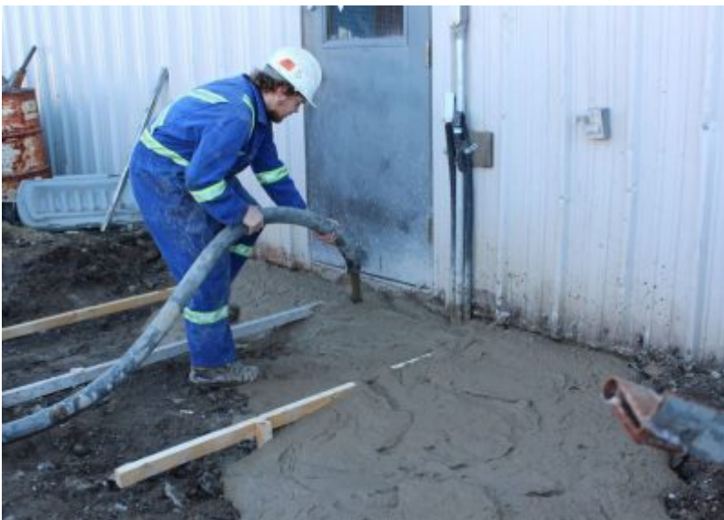
Component Concrete Pad Installation
