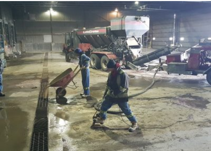
Mudjacking Concrete Roadway
