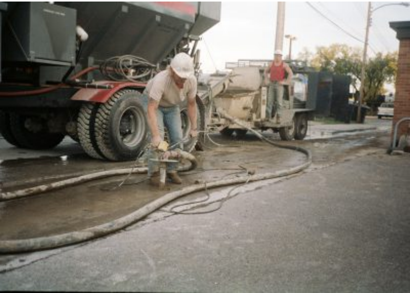
Mudjacking Concrete Roadway
