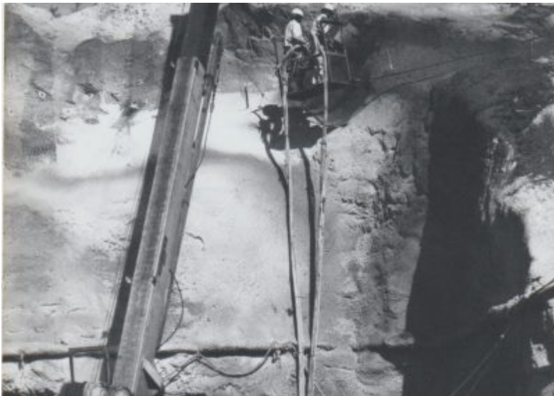
Flin Flon Trout Lake Mine Rock Stabilization
