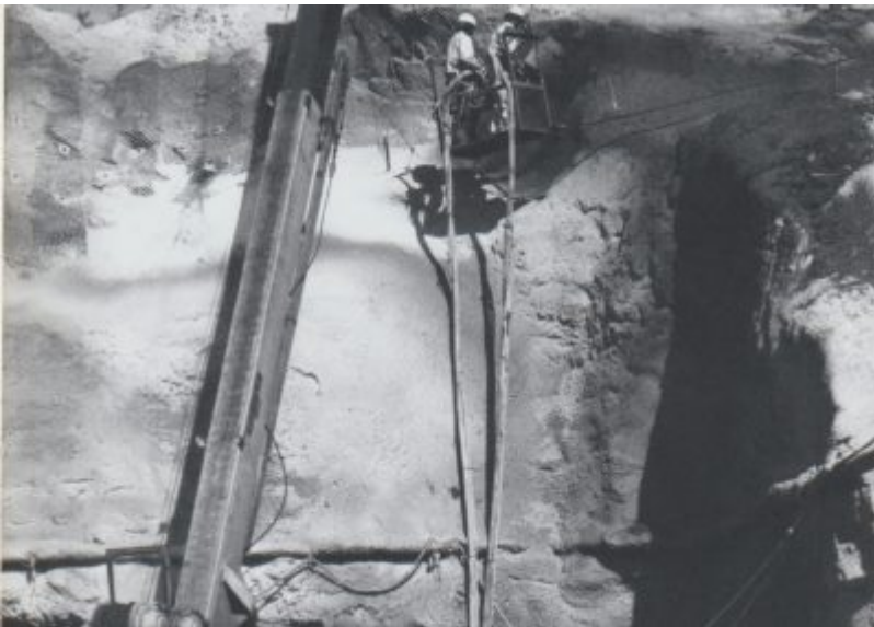
Flin Flon Trout Lake Mine Rock Stabilization
